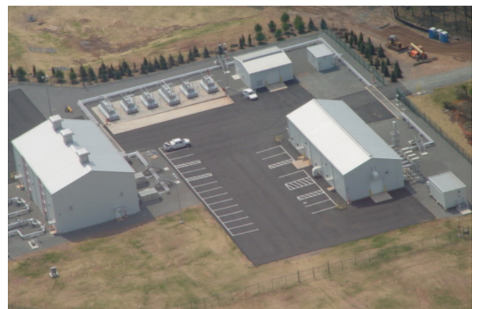
Typical natural gas compressor station.
